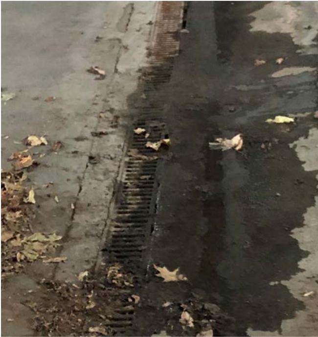
*The previous metal drain here is corroded, which left standing water on the surface.*
