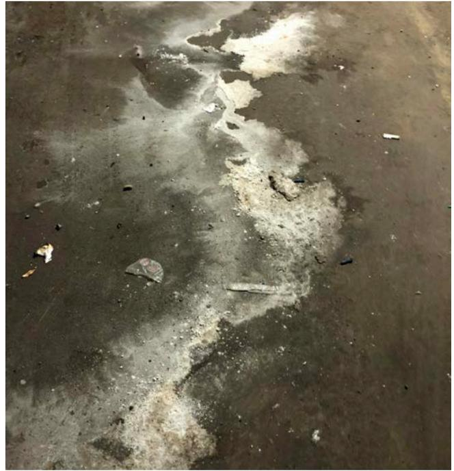
*Another sign of water damage and deterioration is efflorescence, an often-white powdery substance that appears on the slab's surface.*
