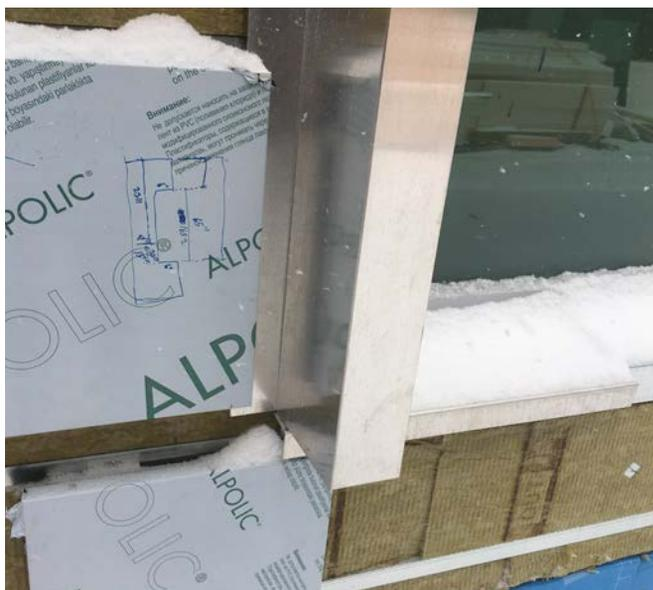
*A mock-up of sun-shade elements supported on a thermally broken cladding support system.*
