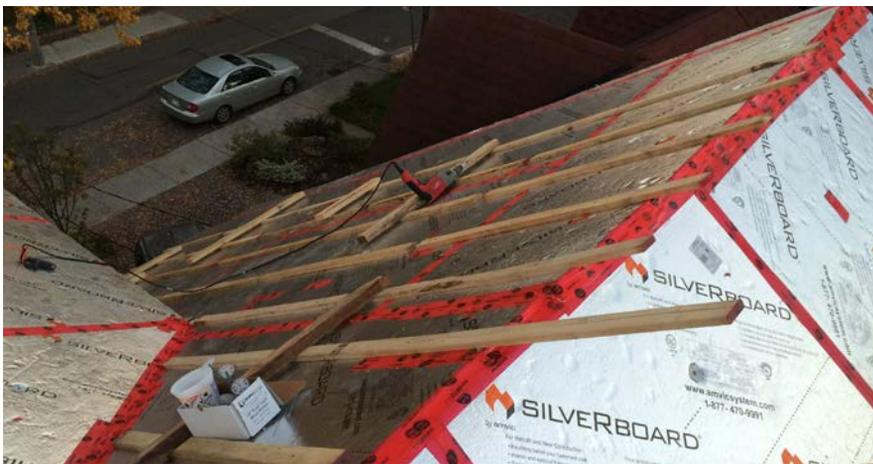
Foil-faced insulation seams taped to provide a continuous water control layer, along with one-by-three wood strapping over-top and screwed to the structure. Two inches of foil-faced EPS insulation over five inches of GPS insulation with staggered seams over the roof structure were then installed.
