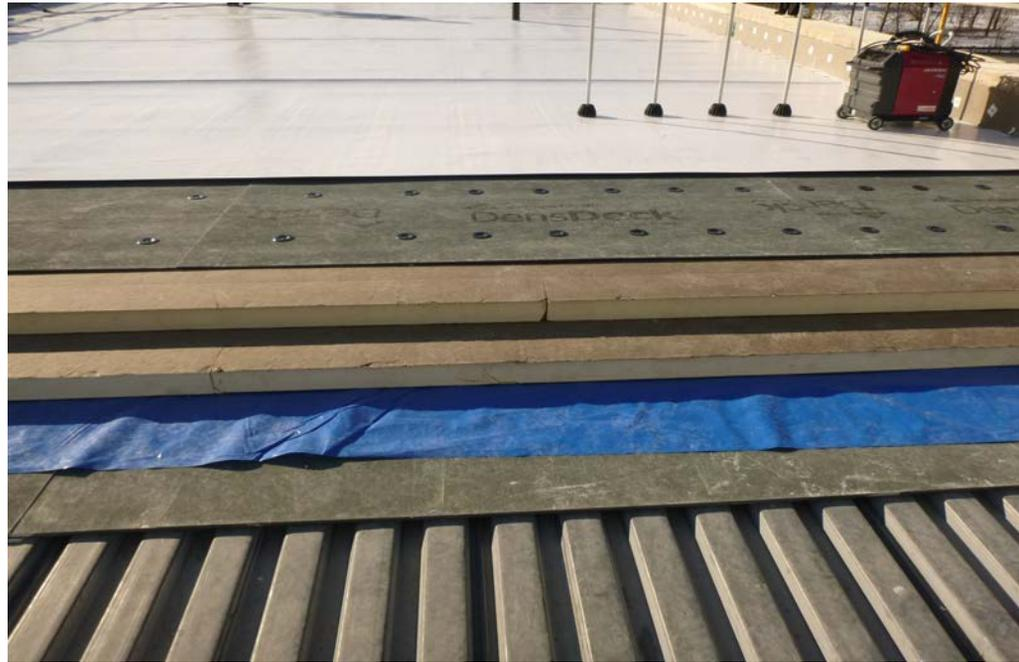
*Layers of a typical conventional roof.*
