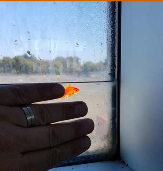
Water retained within an insulating glass unit is a near-sure sign of drainage problems. Okay, the fish was added in Photoshop, but wouldn't that be cool?
