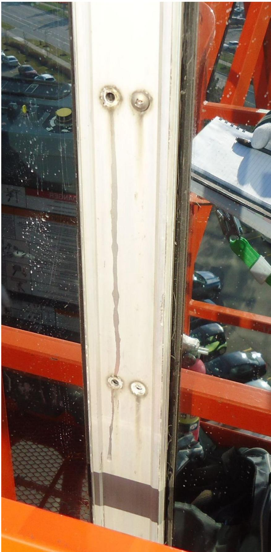
*Retained water trickled from screw holes when backed-off. A little more love and attention to drainage would have prevented these tears.*
