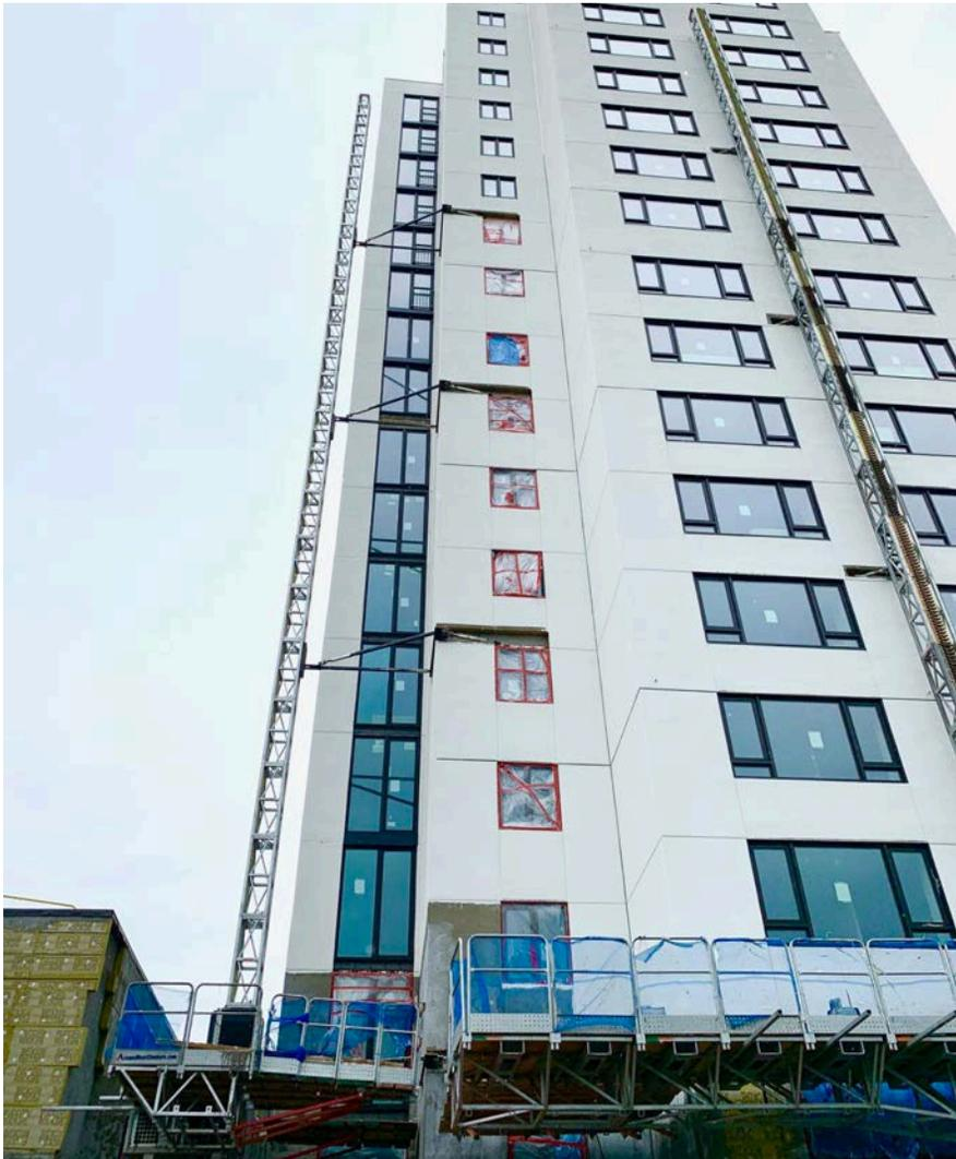
The retrofit underway, featuring the DuROCK PUCSS NC EIFS system with ROCKWOOL stone wool. The system creates the new, white exterior and contributes to the tight and super-insulated building envelope. Photo credit: ERA Architects
