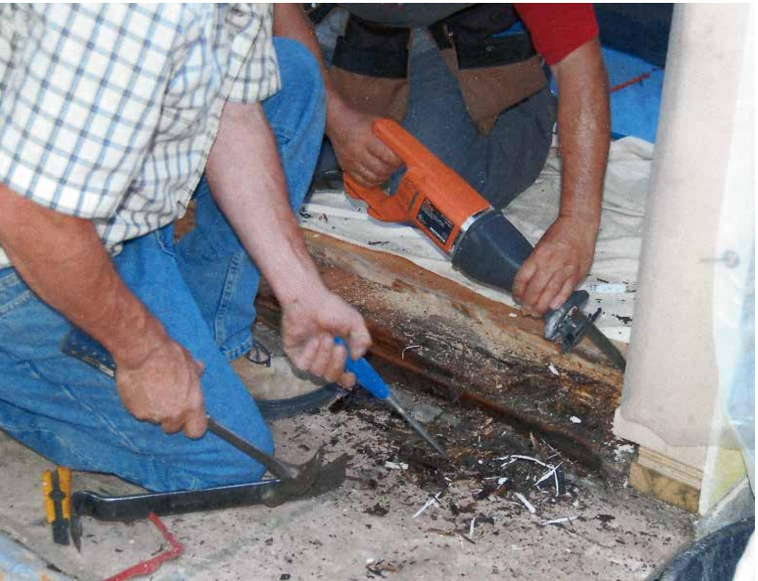
*Failure of face-sealed EIFS led to structural damage inside the wall of this five-year-old custom-built Ontario house (and others), which was later completely re-clad. Photo provided by Pro-Demnity Insurance Company.*
