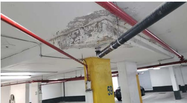
*A concrete ledge beam supporting an intermediate slab experiencing delaminated concrete due to premature failure of the preformed expansion joint installed less than 10 years ago.*
