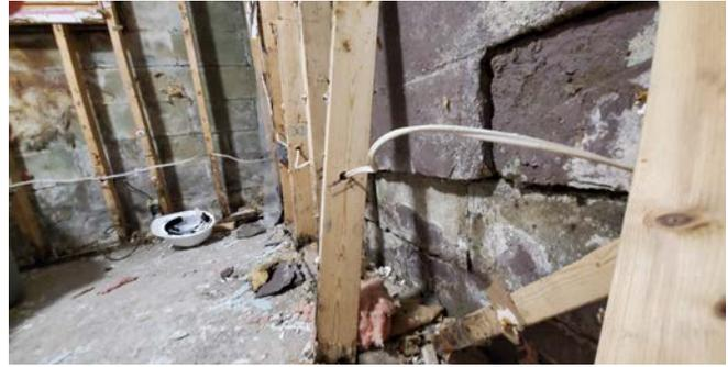
During renovations to a 98-year-old detached house, a contractor discovered major sub-floor damage caused by water penetration from the exterior concrete block foundation wall. The wall was protruding 50 to 75mm out of plane, likely from frost.
