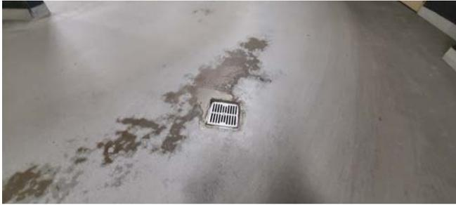
Localized repairs and replacement of worn and debonded membranes should be addressed as part of a maintenance plan to avoid leaving the concrete unprotected and exposed to water and de-icing salt, which can lead to corrosion of the embedded reinforcing steel.
