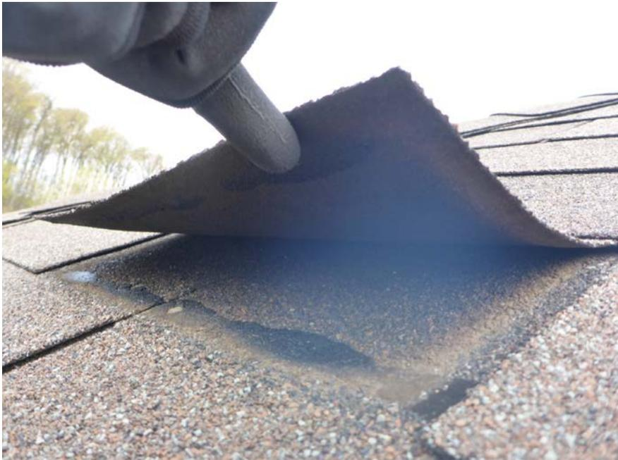
*A view of the adhesive strip between three-tab shingles not engaged and properly bonded.*
