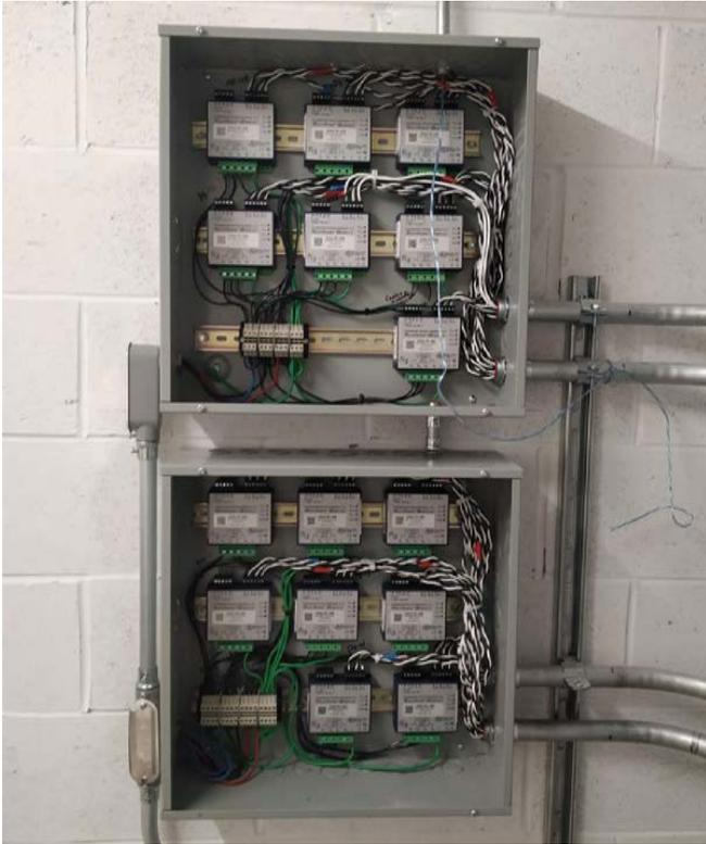
*Electrical submetering installed in one of the study buildings.*
