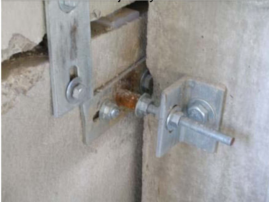
Inside view of joint yet to be caulked
