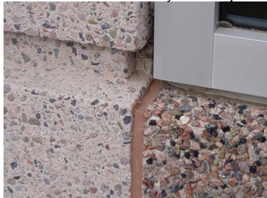
Outside view of neatly caulked joint
